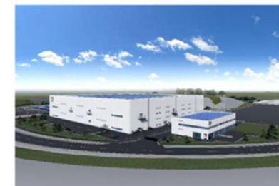
Tomiya new factory (Under construction)
